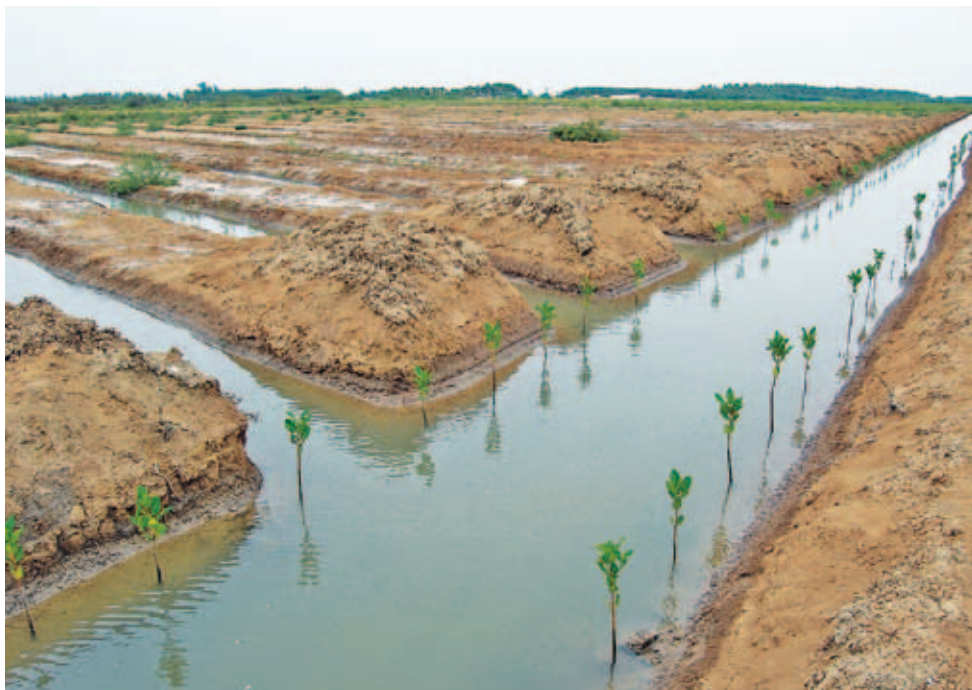
Figure 3 Fishbone canal system developed to facilitate free tidal flushing of saline blanks. Photo © MSSRF.
